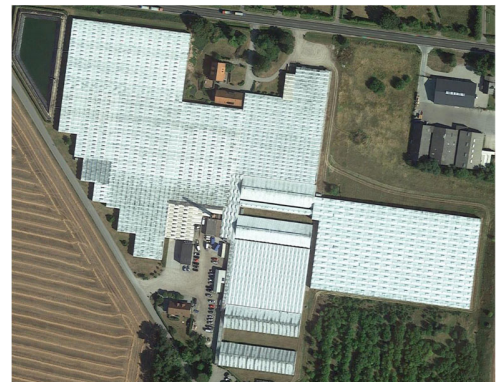
Fig. 3. Overhead of the industrial greenhouse facility
