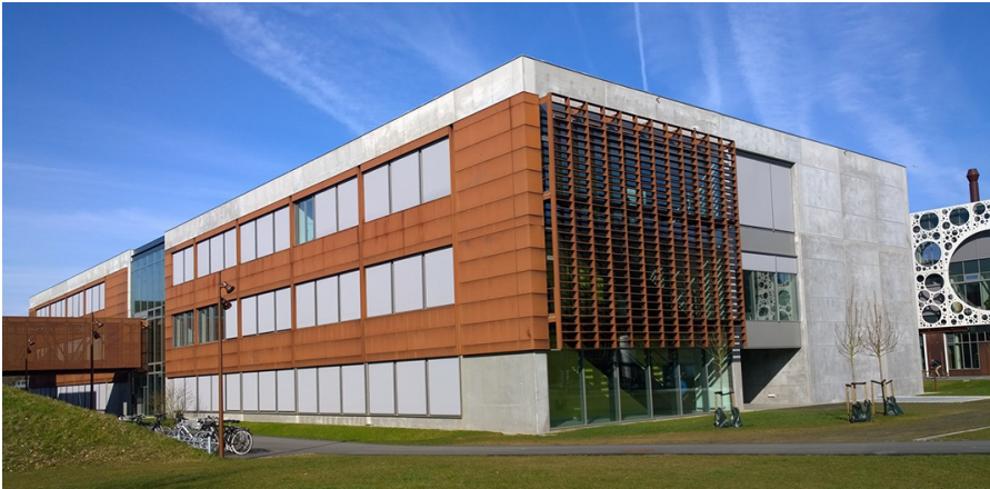
Figure 14.13: The University of Southern Denmark OU 44 Living Lab used for the Brick Model and for the data used in the OccuRE services.
